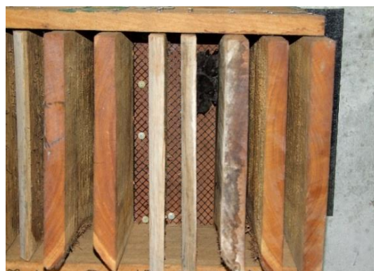
Figure 8. a) Bat boxes installed in culverts over a wetland have been successful in attracting the Southern Myotis, a microbat species listed as vulnerable in NSW; b) the box is large with many chambers to accommodate different group sizes; c) the vertical chambers of varying width are flanked by timber of varying thickness
