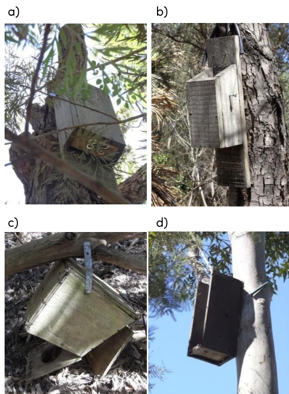
Figure 3. Common problems with artificial hollows from the Authority's first nest and roost box project; a) bat box entrance obscured by branches; b) bat box attached to a small branch, with lid missing; c) marine ply possum box with poor attachment and in disrepair; d) marine ply bird box with missing panels; attachment does not allow for tree growth
