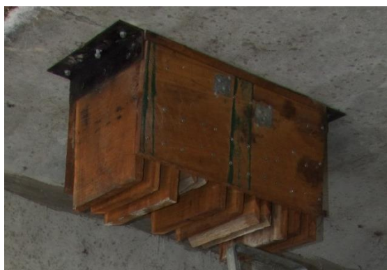
Figure 8. a) Bat boxes installed in culverts over a wetland have been successful in attracting the Southern Myotis, a microbat species listed as vulnerable in NSW; b) the box is large with many chambers to accommodate different group sizes; c) the vertical chambers of varying width are flanked by timber of varying thickness
